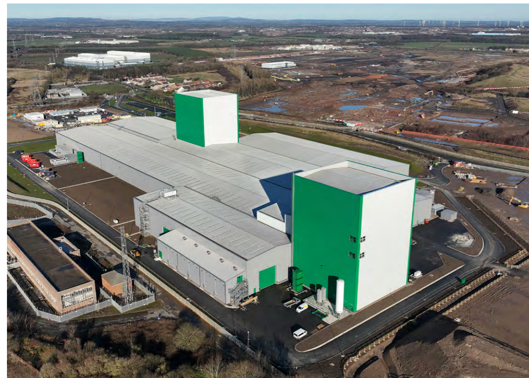
JDR Cable Factory Cambois
